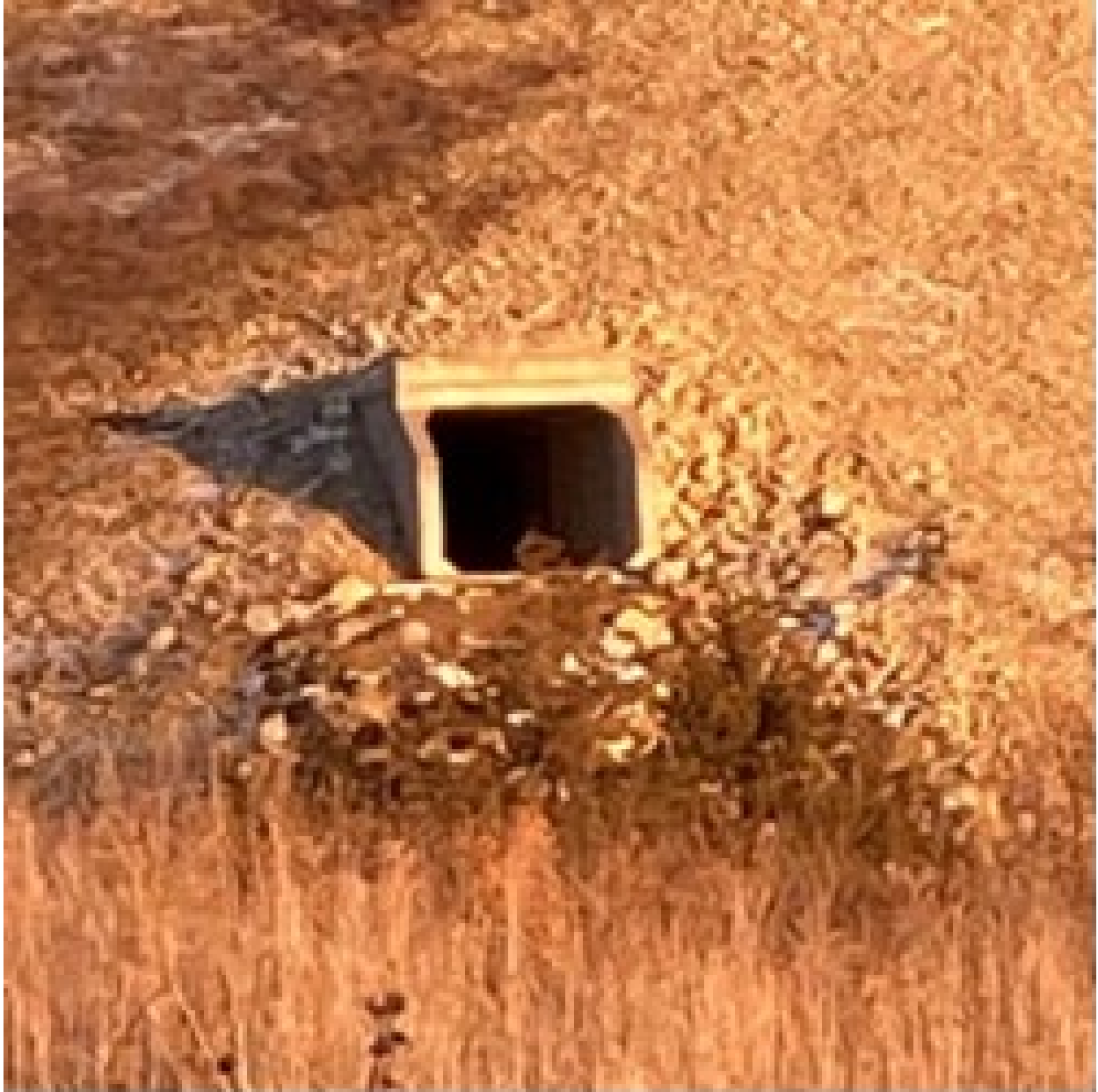
Figure 8 A. Examples of culverts, which can be many shapes and sizes and found in a variety of locations. Example A is a very large box culvert running underneath an interstate. (Photo credit: Christy-Ann Archuleta).
